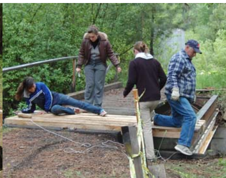
Attaching the planks
